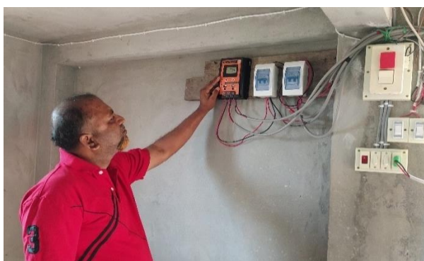
c. SHS at Kolapara, Patuakhali
